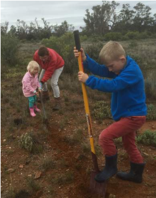
Jack and Ruby erecting a pitline fence assisted by Helen
