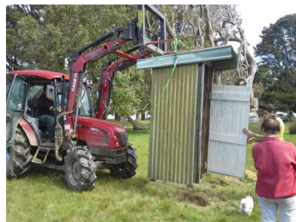
Restoring the longdrop at Minnowarra
