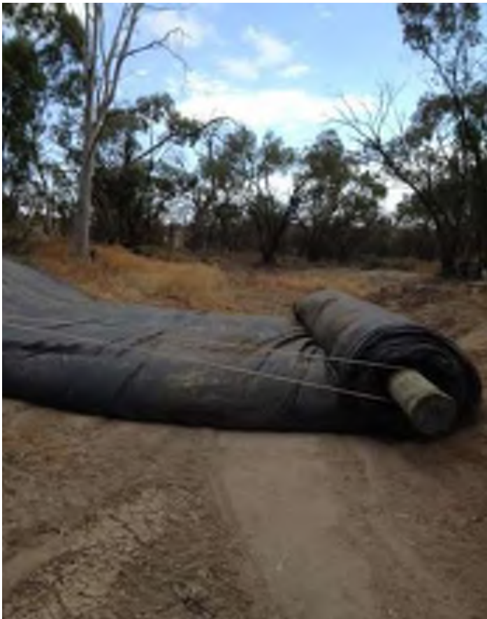
AquaDam partially rolled out . Photo: Peter Forward
