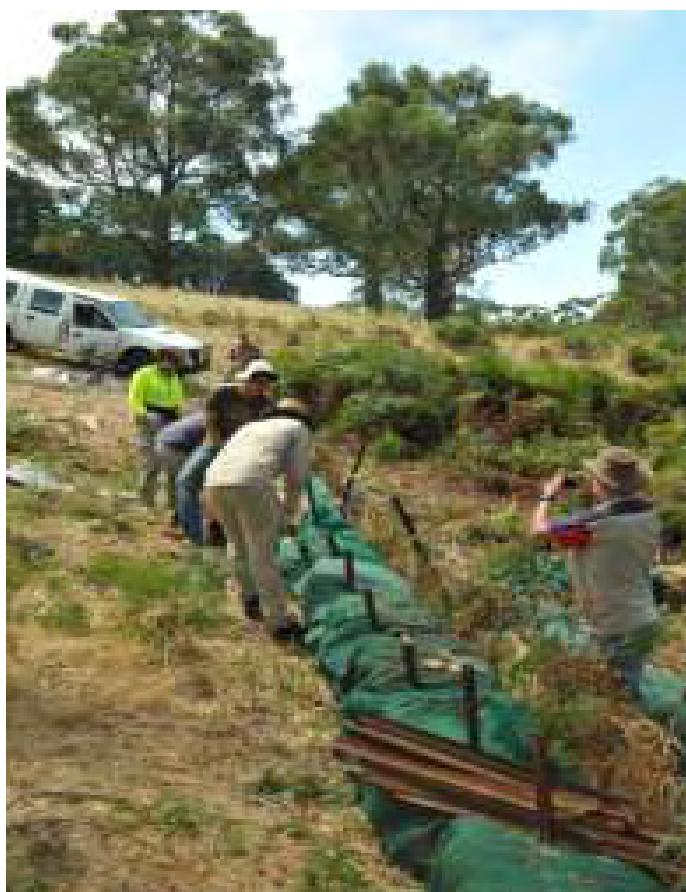
**Figure 8:** Erosion control is achieved by slowing and dispersing water flow using hay bales, wrapped in shadecloth, held in place by old droppers.
