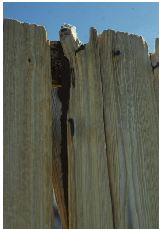
Two views of the structure of the Absolute Magnetic Hut taken in 1985 showing serious timber erosion over more than 70 years. The copper nails can also be seen in the lower photo.
